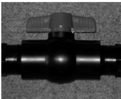
Valve in the open position Solar heating is OFF ( not heating ) Fig 1a
