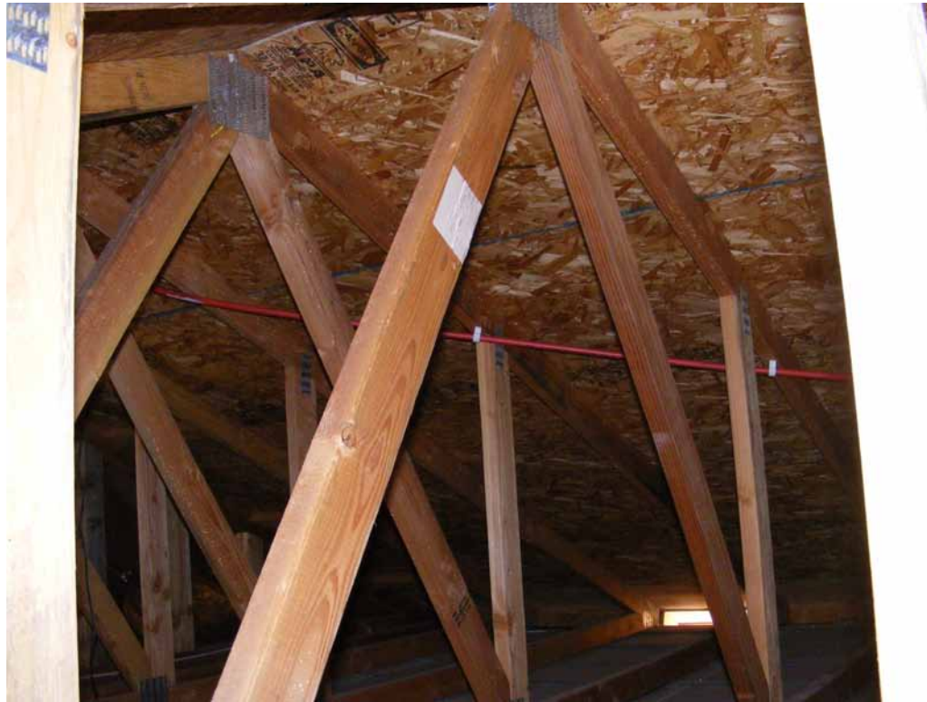
Example Tubing Run From Upper Roof Jack
